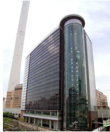
Kenko Plaza Toshima health centre, next to the cleaning plant
