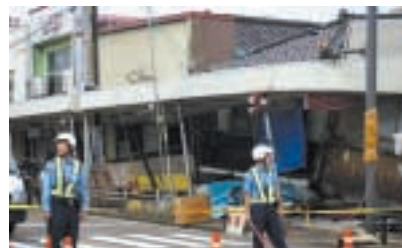
The aftermath of the July earthquake in Niigata.
