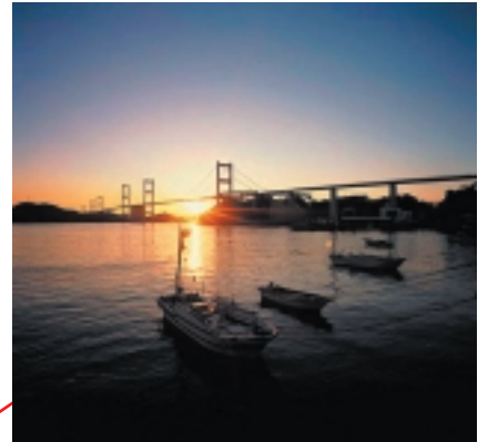
Imaban Itoyama Bridge, Ebime Prefecture
