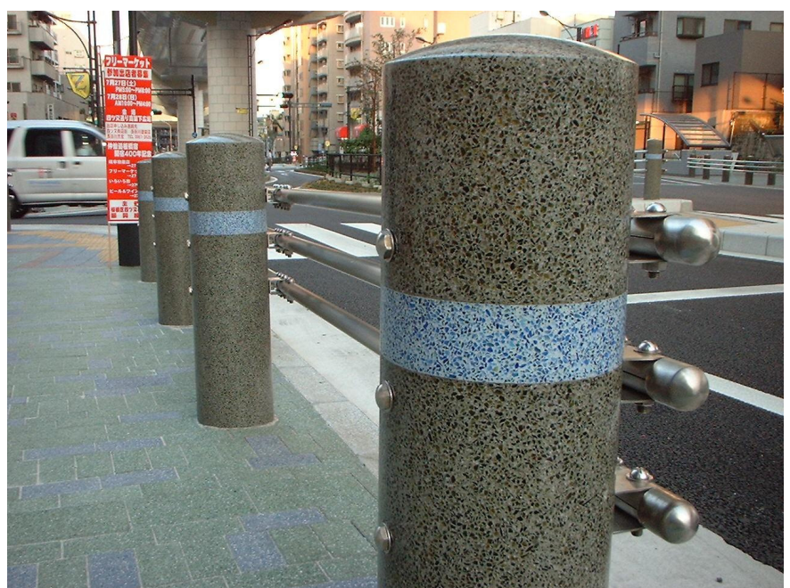
Above: Bollard made from glass
