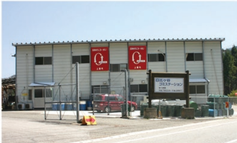
Above: the Kamikatsu recycling station.
