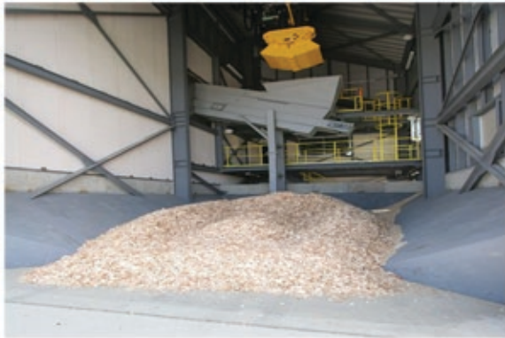
Above: inside the woody biomass gasification power plant
